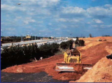
Advancing fill on
