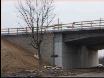
retaining walls & bridge wings
