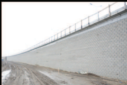
retaining walls & bridge wings
